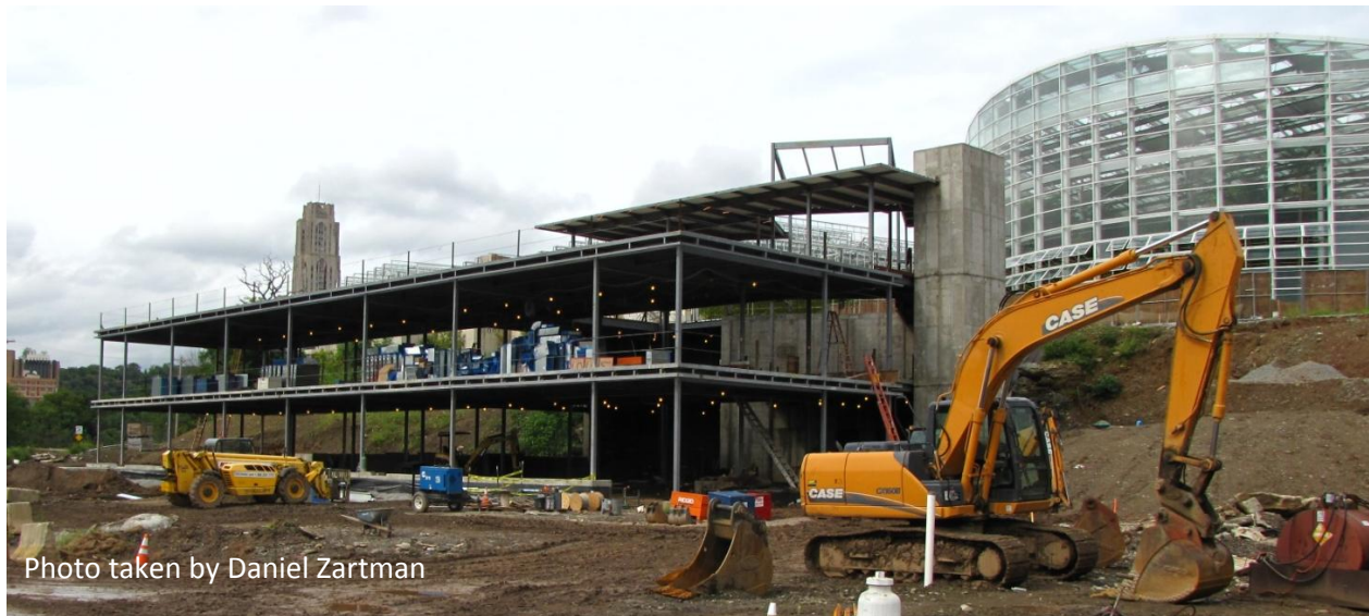
Figure 3 - Concrete and steel superstructure taken September 7, 2011.
